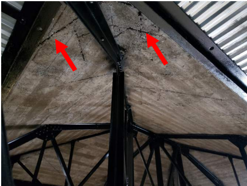
Figure 6. Underside of dome cap. The dark lines (red arrows) are embedded wood that Pishny noted have little to no concrete cover.
