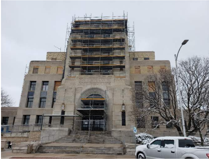
Figure 1. South elevation of the Reno County Courthouse.
