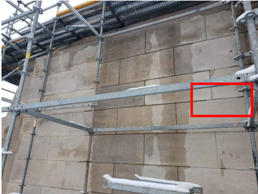
Figure 7. East elevation of the tower. See Figure 8 for an enlarged image of the "half-moon" stone crack boxed in red.
